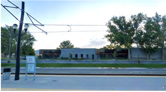
FIGURE 8 WEST (LEFT) AND EAST (RIGHT) VIEW FROM RIVER TRAIL STATION
