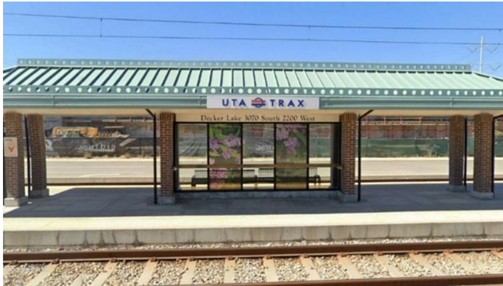
Figure 56: Decker Lake Station Shelter Window Art
